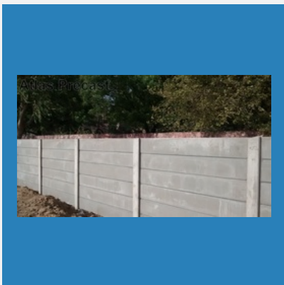
Precast Compound Wall
