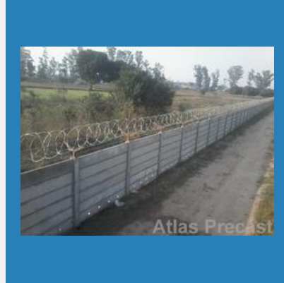
Industrial Compound Wall
