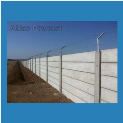
Security Boundary Wall
