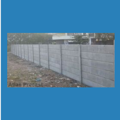
Concrete Precast Boundary Wall
