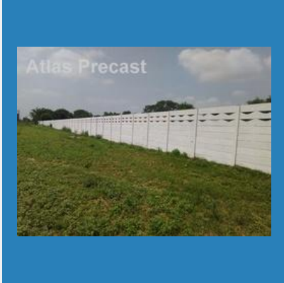
Precast Compound Wall
